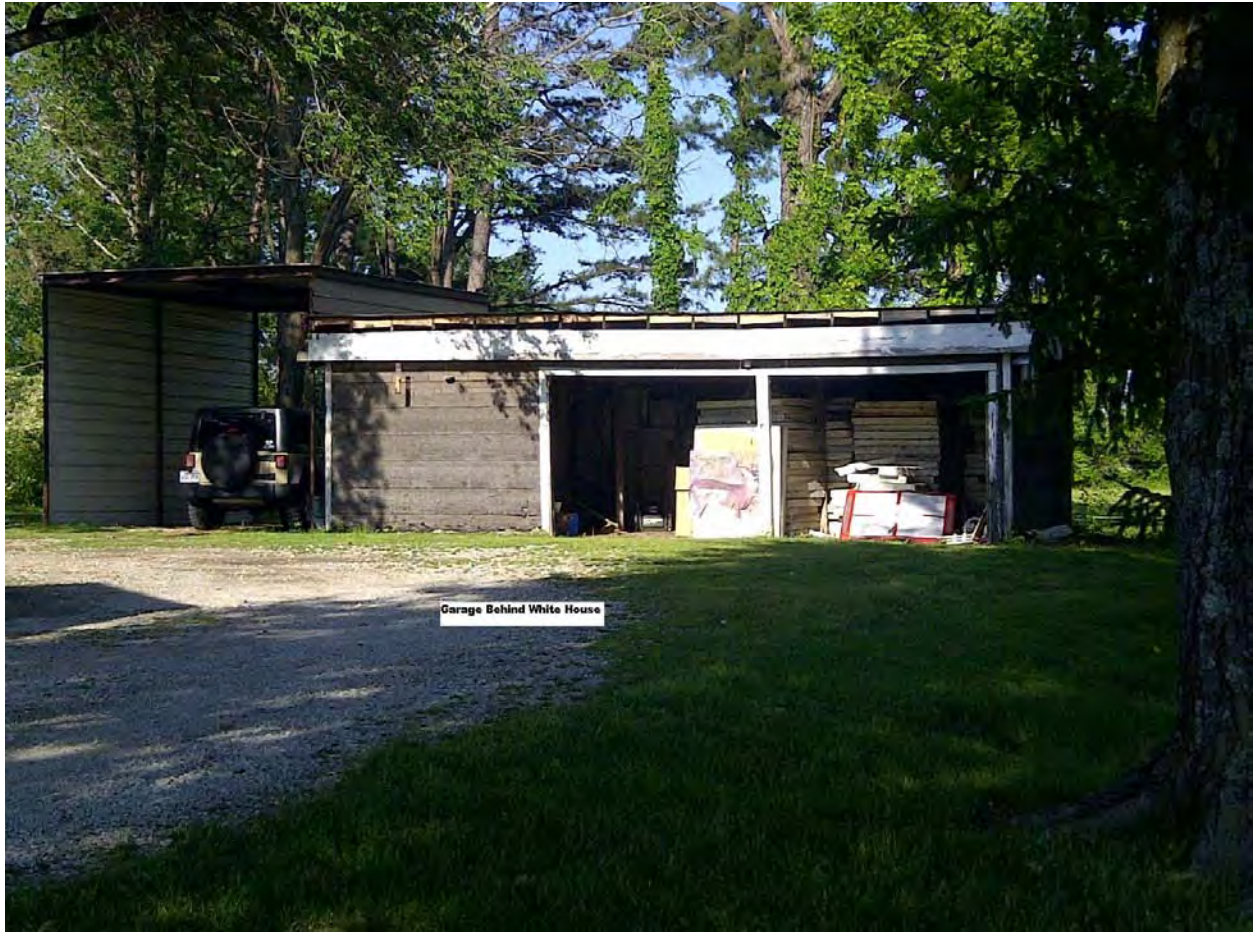
Figure 15 - 2258 N. 2nd St., Out Building (Small Garage)
