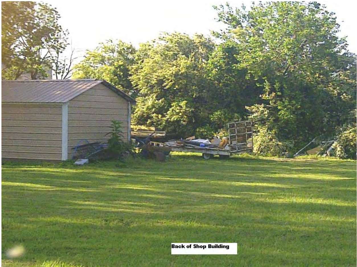
Figure 12 - 2256 N. 2nd St., Back of Shop Building
