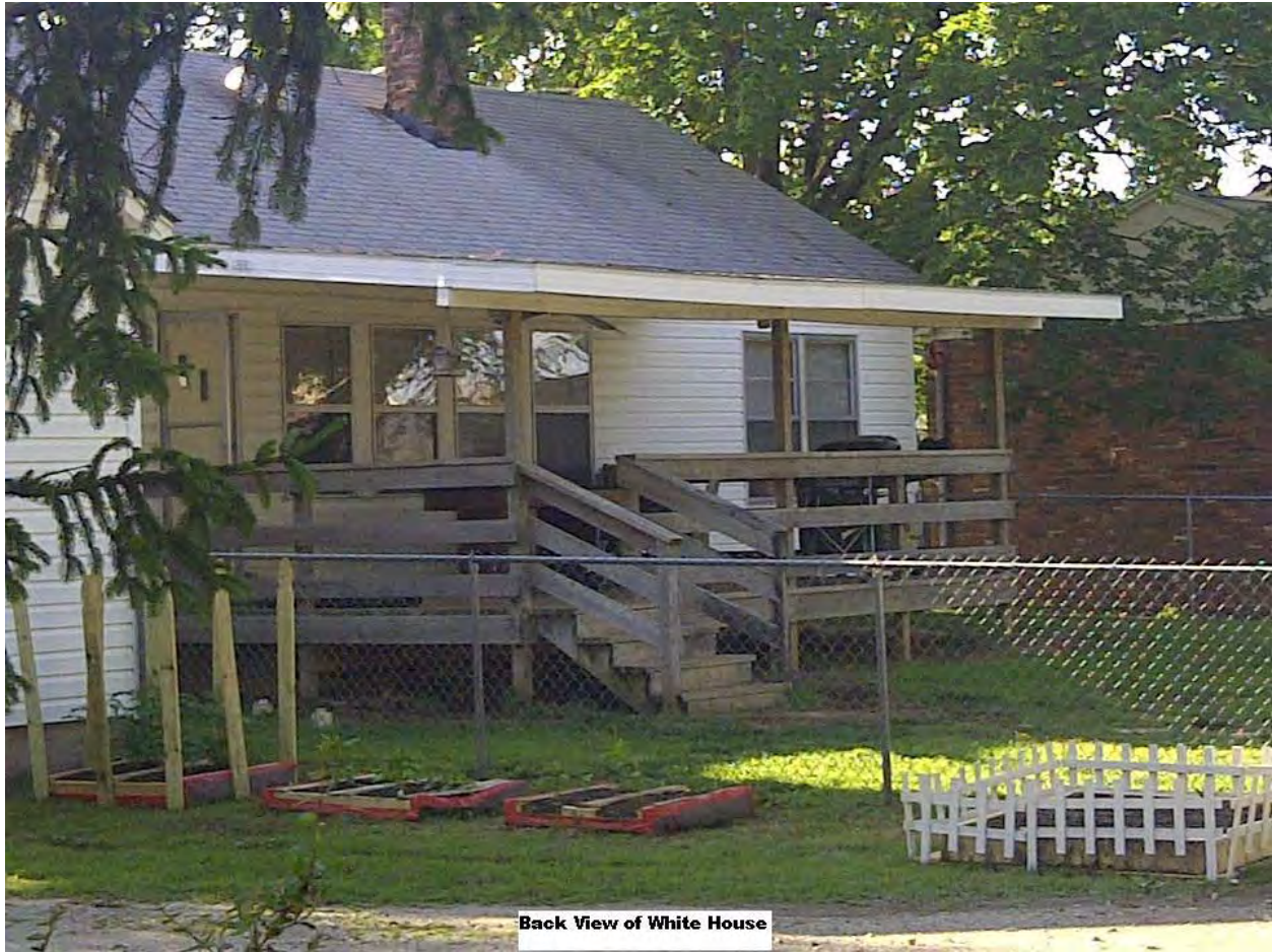
Figure 14 - 2258 N. 2nd St., Back View of Residence
