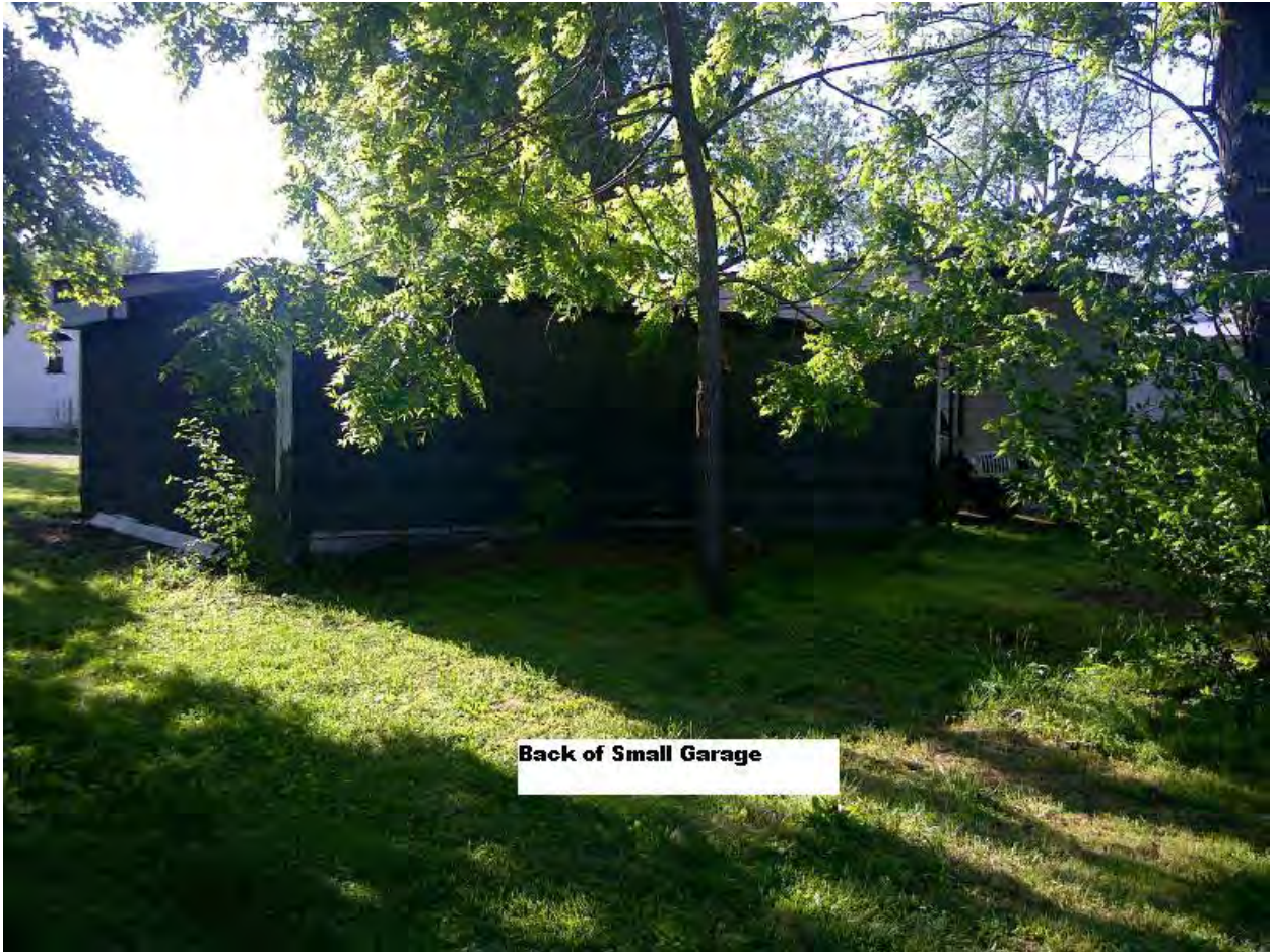
Figure 16 - 2258 N. 2nd St., Back of Small Garage (Out Building)
