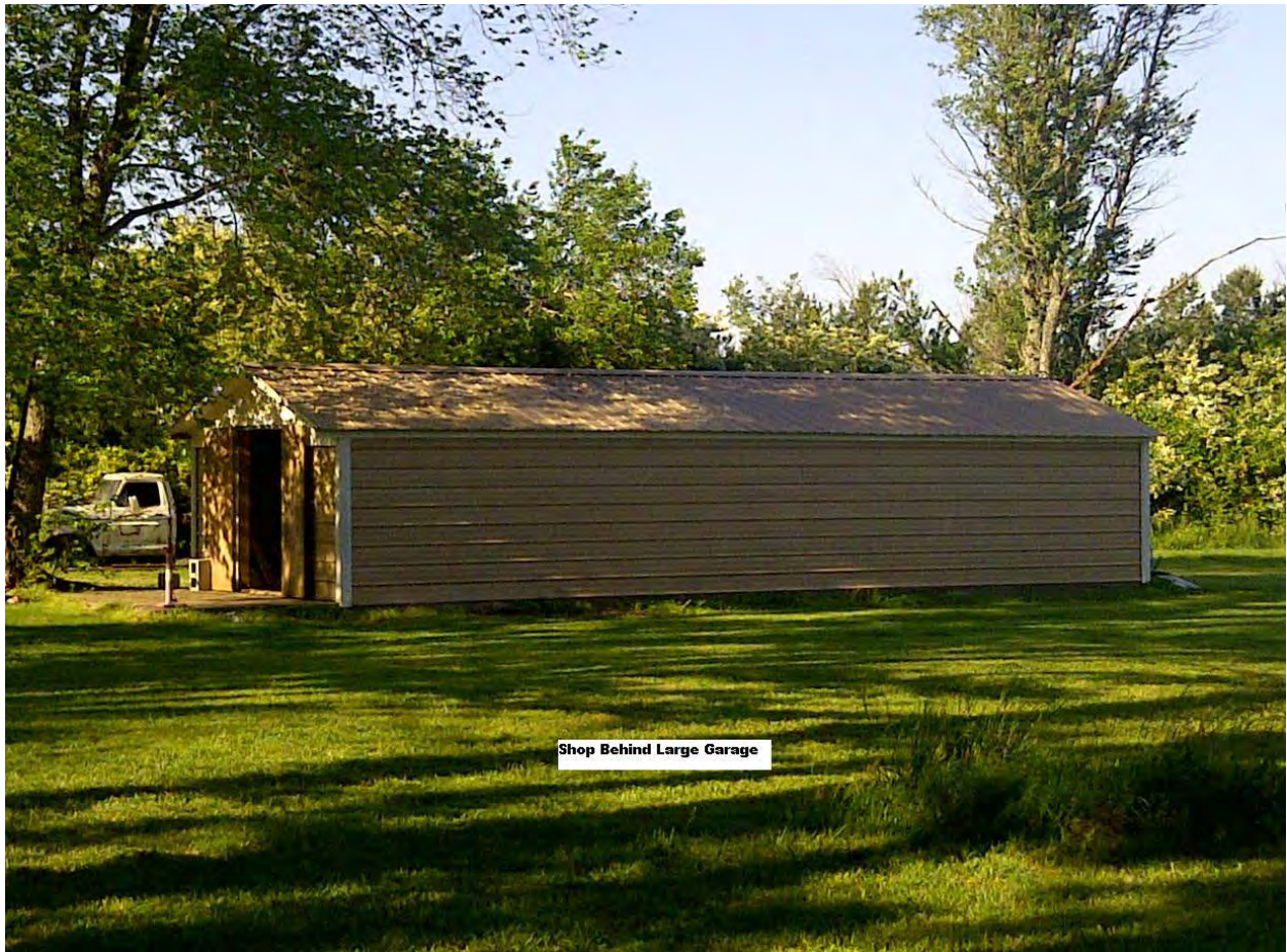
Figure 11 - 2256 N. 2nd St., Shop Building
